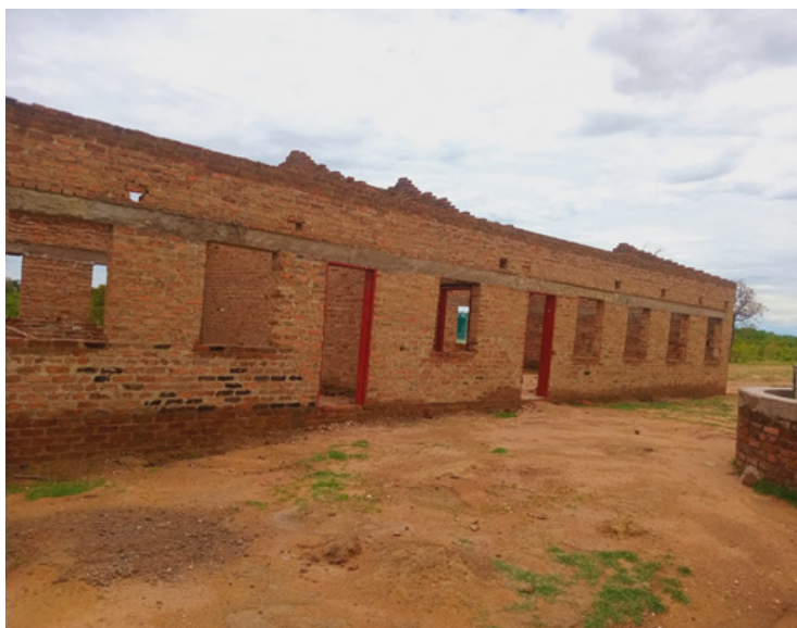
Construction of Zvimhonja Secondary Funded by Garden Project
