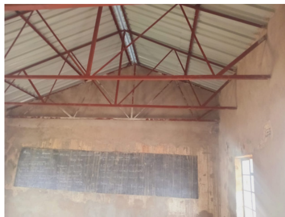
Denderedzi Roof Renovations
