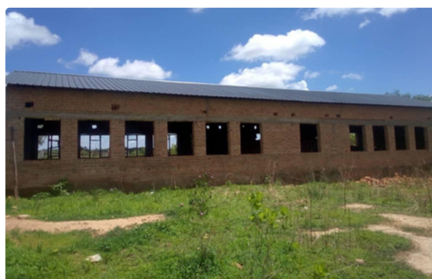
Musukwi - TTI Construction Progress
