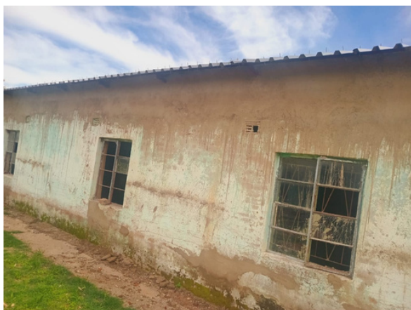
Denderedzi Pri Block Wall Ronovations
